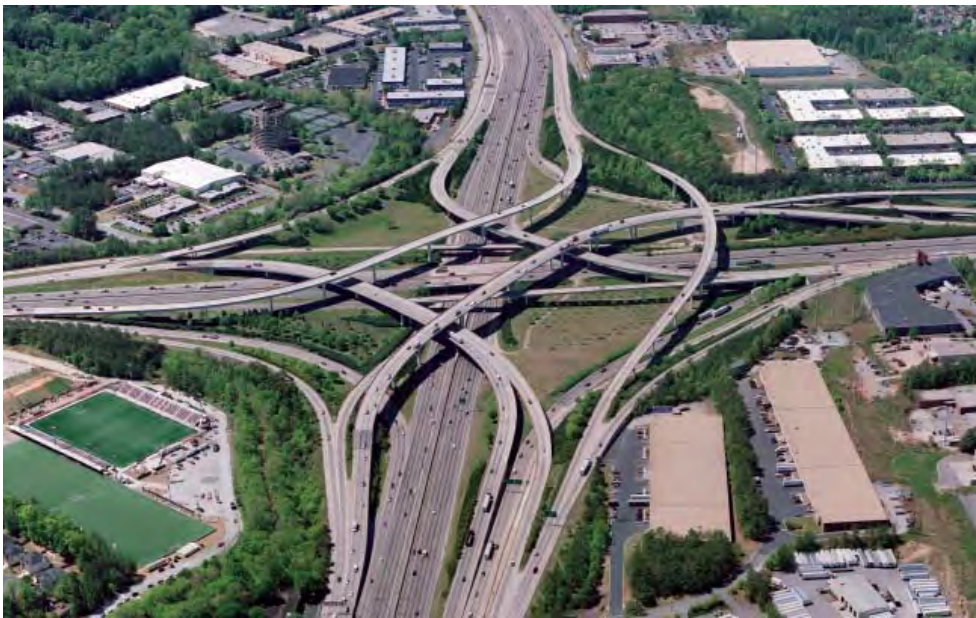
Figure 10-36. Four-Level Directional Interchange
