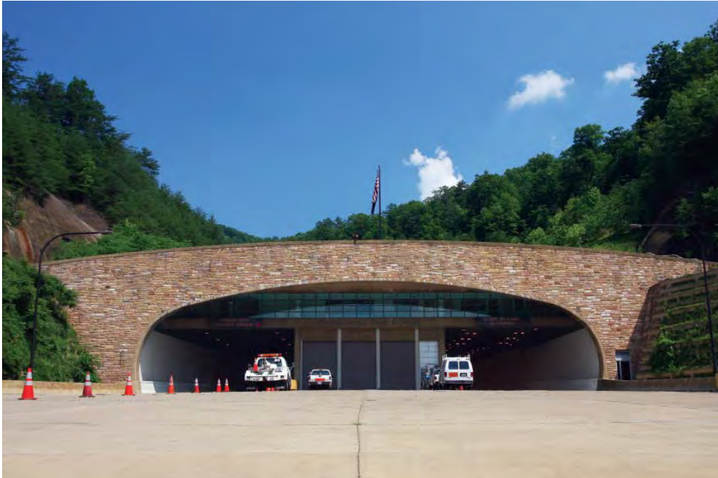
Figure 4-16. Entrance to a Freeway Tunnel
