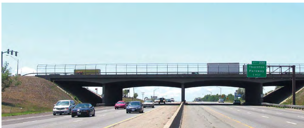
Figure 10-4. Typical Grade Separation Structure with Open-End Span
