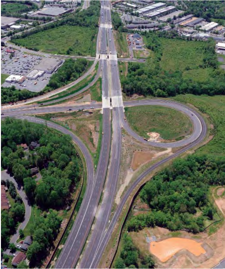
Figure 10-14. Trumpet Freeway-to-Freeway Interchange
