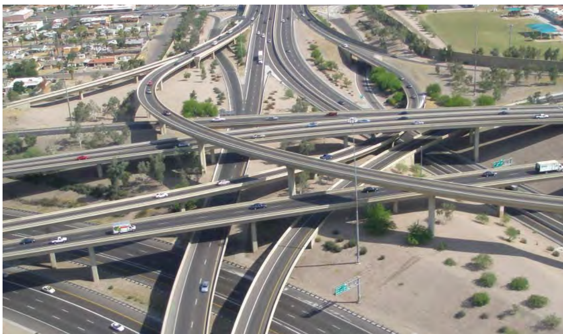
Figure 10-37. Four-Level Directional Interchange
