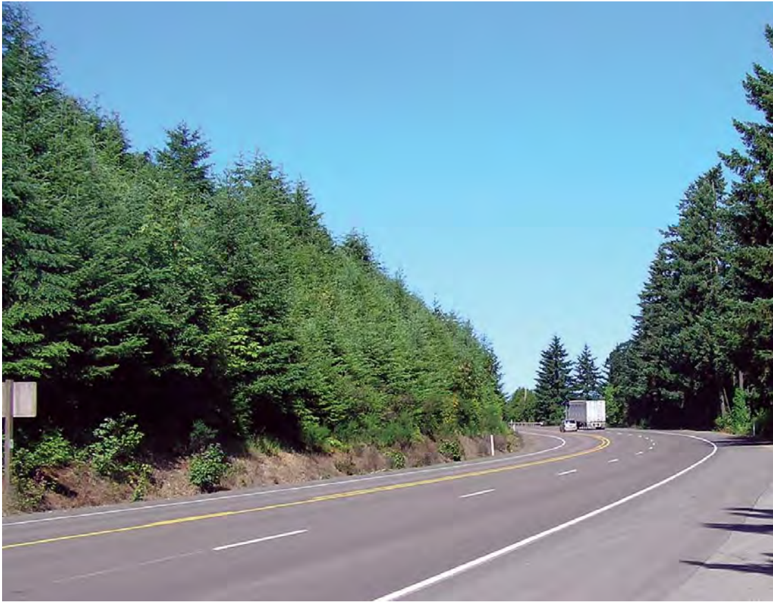
Figure 7-1. Climbing Lane on Two-Lane Rural Arterial
