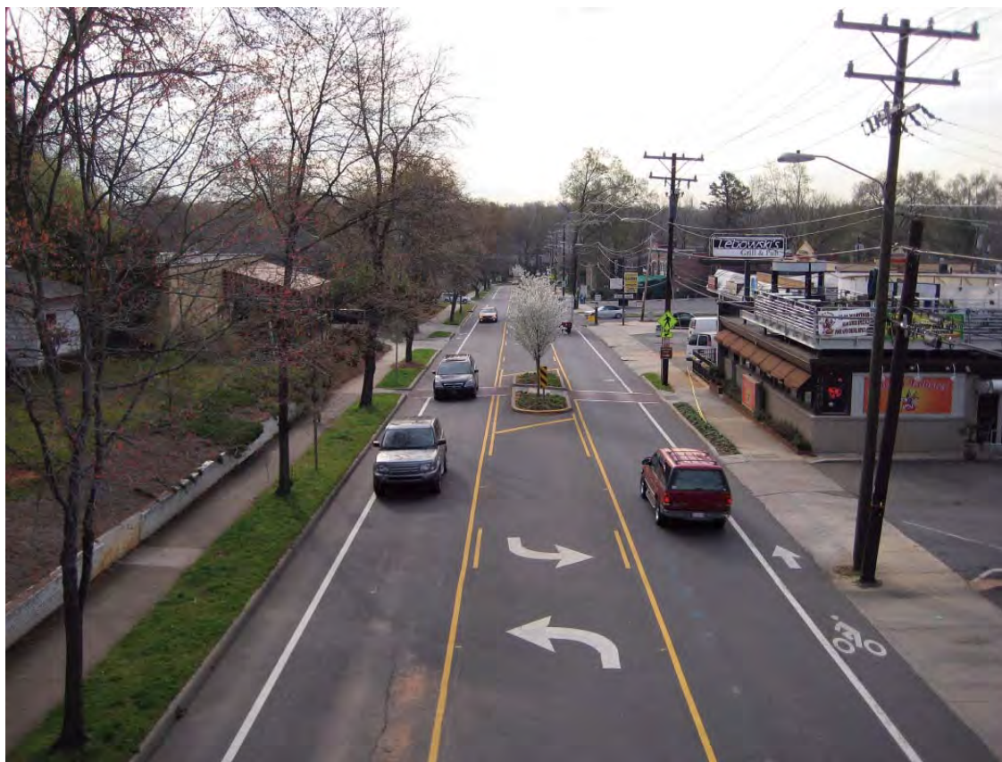
Figure 7-7. Continuous Two-Way Left-Turn Lane
