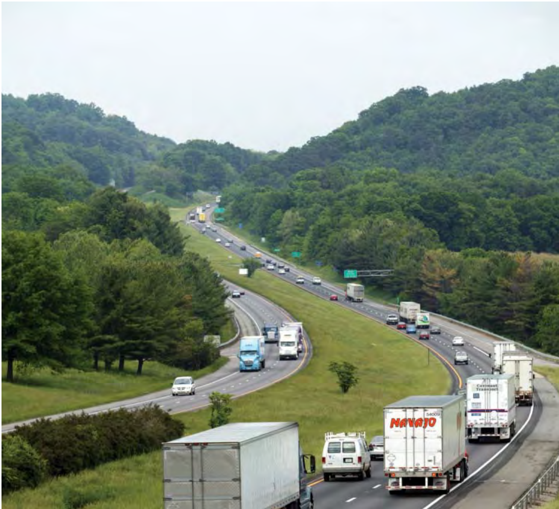
Figure 8-1. Typical Ground-Level Rural Freeway
