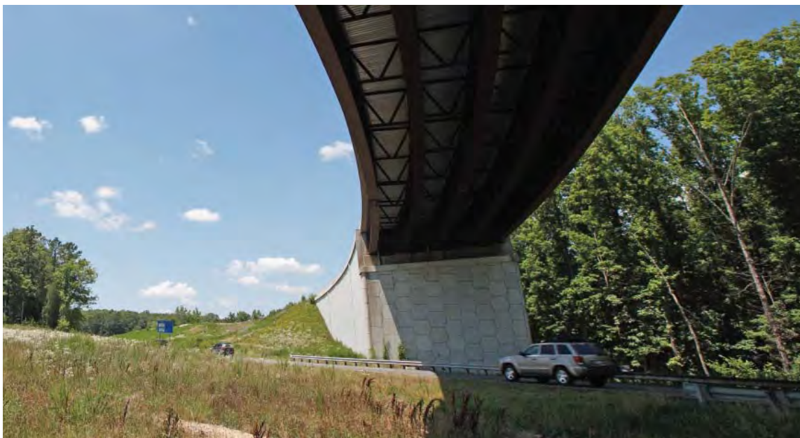
Figure 10-3a. Typical Grade Separation Structures with Closed Abutments
