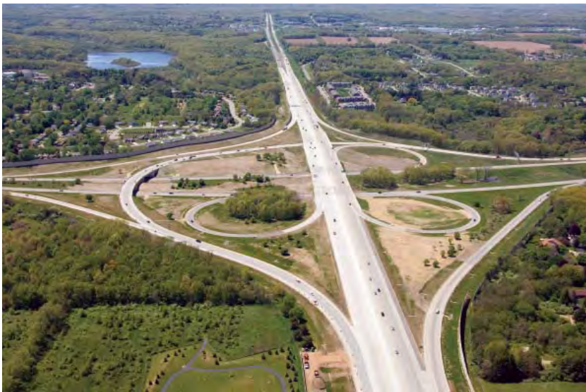
Figure 10-41. Four-Leg Interchange, Cloverleaf with a Semidirect Connection
