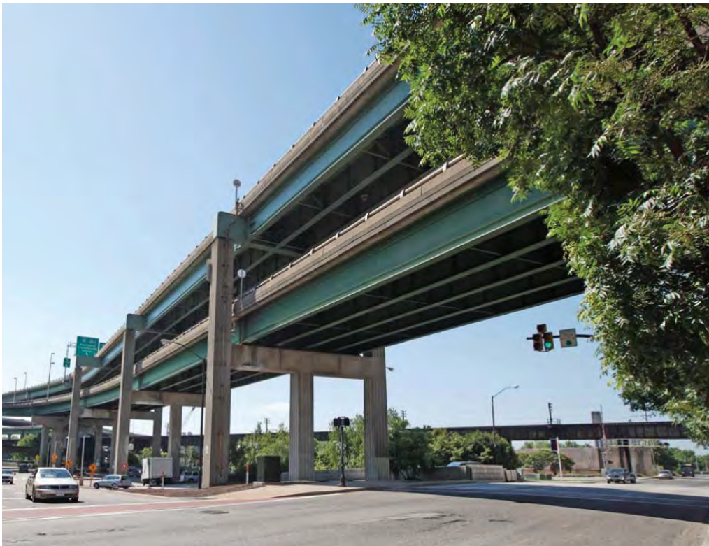
Figure 8-11. Two-Level Viaduct Freeway
