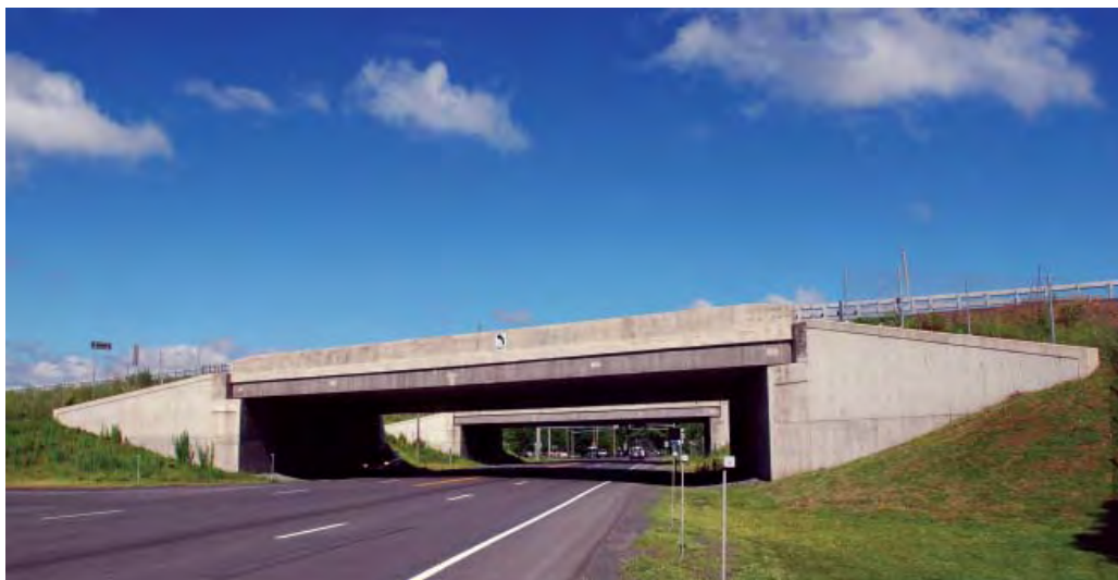
Figure 10-3b. Typical Grade Separation Structures with Closed Abutments
