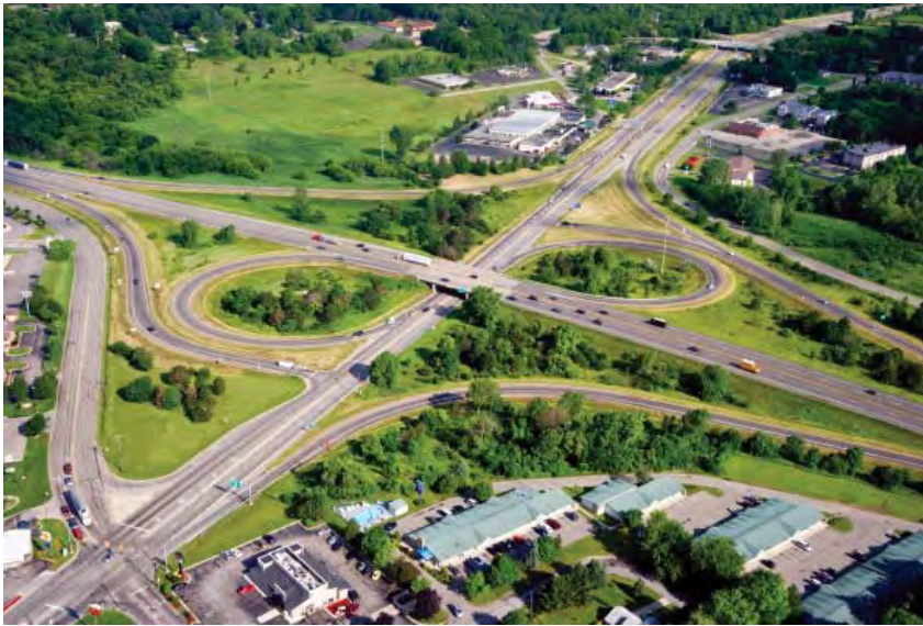
Figure 10-27. Partial Cloverleaf Interchange
