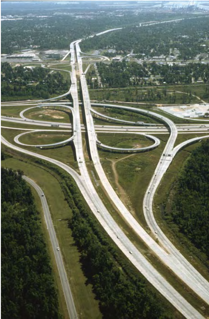
Figure 10-42. Cloverleaf Interchange with Semidirect Connection
