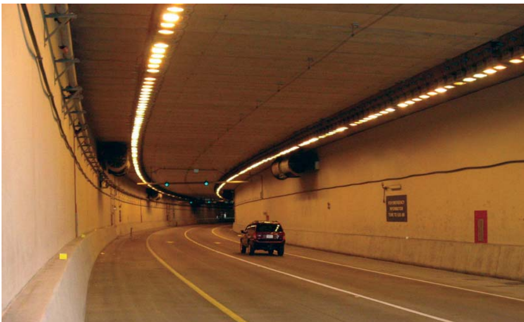
Figure 4-17. Interior of a Two-Lane Directional Tunnel
