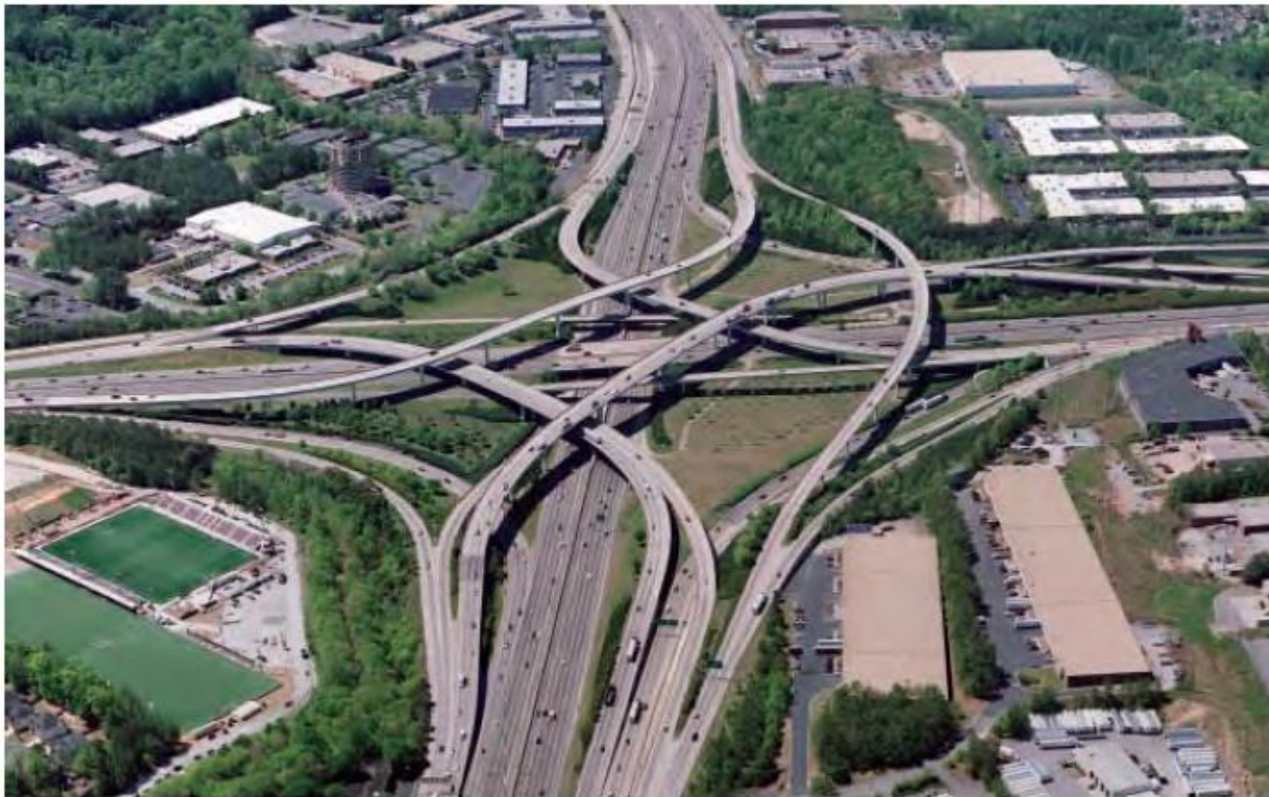
Figure 10-36. Four-Level Directional Interchange
