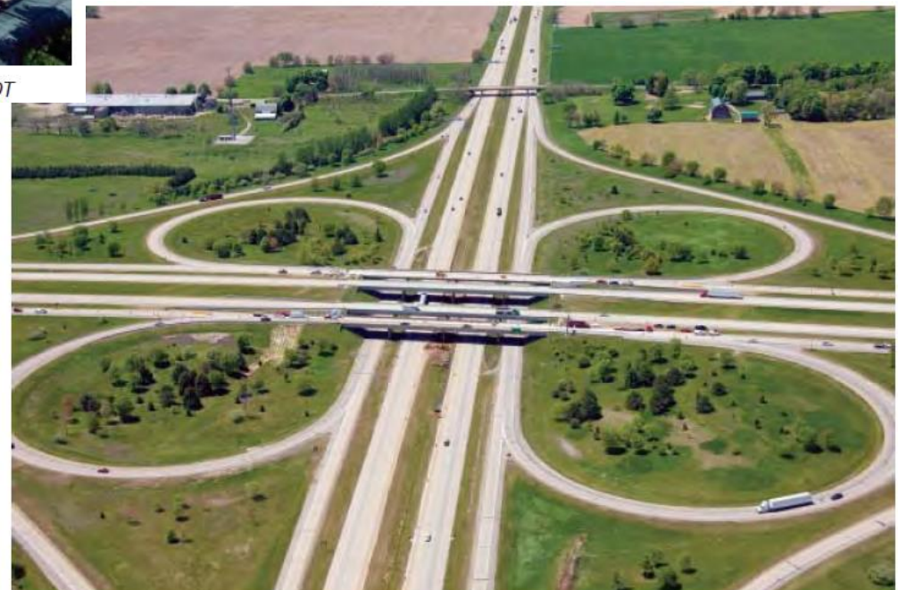
Figure 10-28. Four-Leg Interchange, Cloverleaf with Collector-Distributor Roads
