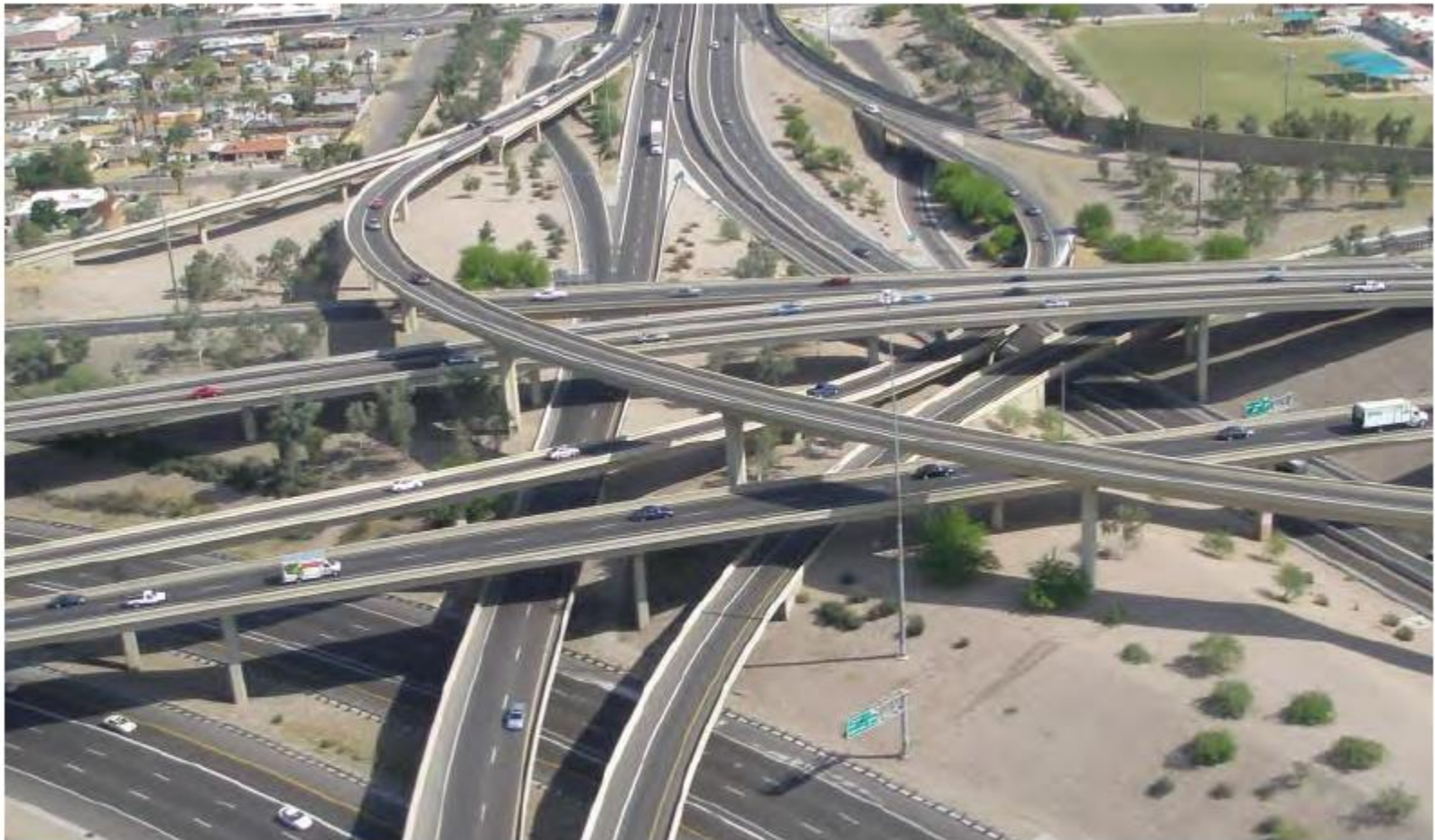
Figure 10-37. Four-Level Directional Interchange
